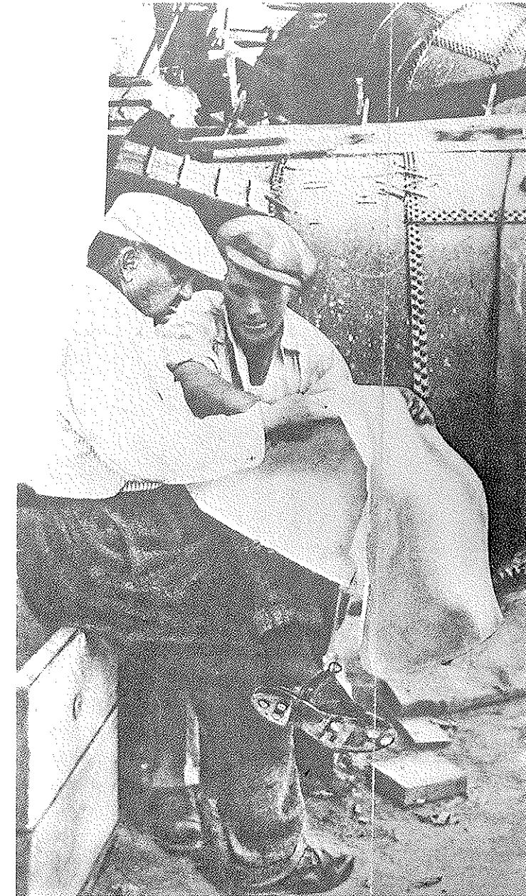
Fig. 6.5 Capitalism Meets Socialism: The image shows the American engineer Hugh Cooper (left) advising a Soviet expert building the Dnieper power plant, by then the world's largest hydroelectric plant. In 1932, the Soviet government awarded Cooper the Order of the Red Banner of Labour. Cooper was hardly the only engineer from the capitalist West who advised the Soviet Union. At that time Soviet administrators were more willing to rely on foreign experts than was the case in later projects to foster industrialization.
