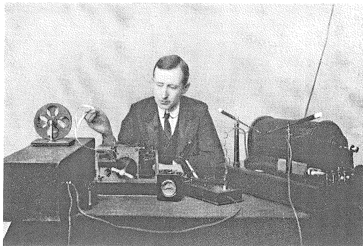
Fig. 5.4 Young Father of Wireless: Based on James Clerk Maxwell's electromagnetic theory of light, the German physicist Heinrich Hertz developed a radio wave transmitter and an antenna receiver. Publications on Hertz's experiments after his death in 1894 sparked young Guglielmo Marconi to realize a practical system for the wireless transmission of telegraph messages. The picture shows Marconi and his technical system that included a spark-producing radio transmitter, a coherer receiver, a telegraph key, and a telegraph register to record messages received in Morse code.
